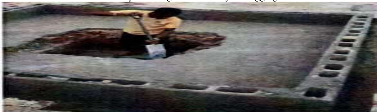
Figure 16: Digging the foundation for the work
