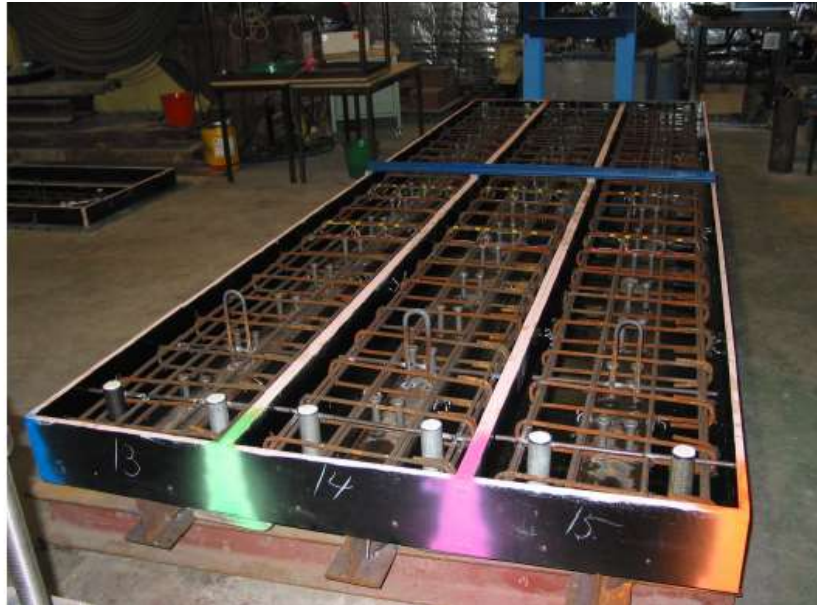
Figure.8 Beam test specimens ready for concrete casting
