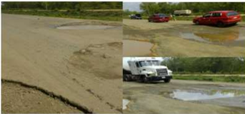
Figure 2. Failed Portion of Itoke-Ajaokuta Expressway.
