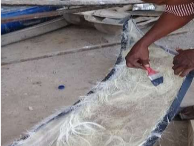
Plate IX: Application of polyester- resin to the fibre
