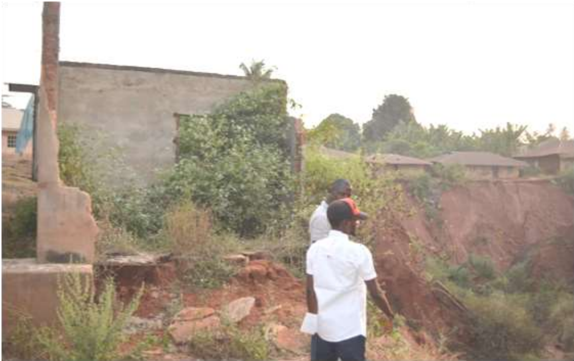
Photo of Ewu Gully Erosion Site Edo Central Showing Abandoned Building
