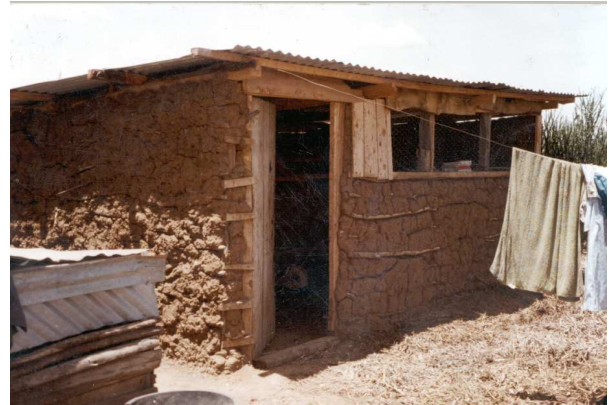
Figure 4.4. A chicken house with iron roofing and mud walls
