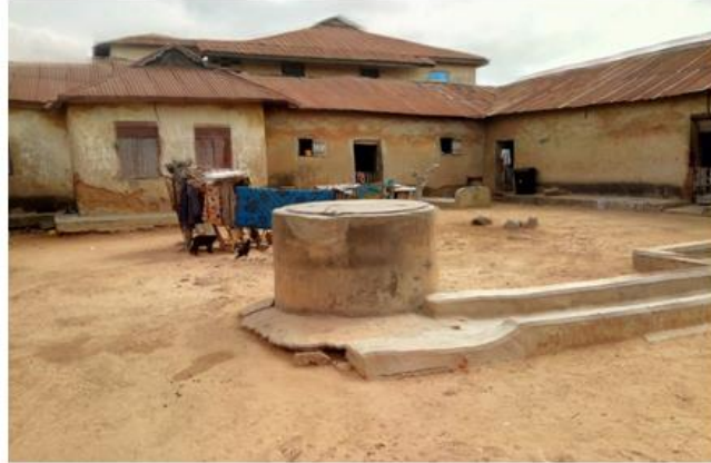
Plate 1: View of a Compound Impluvium
