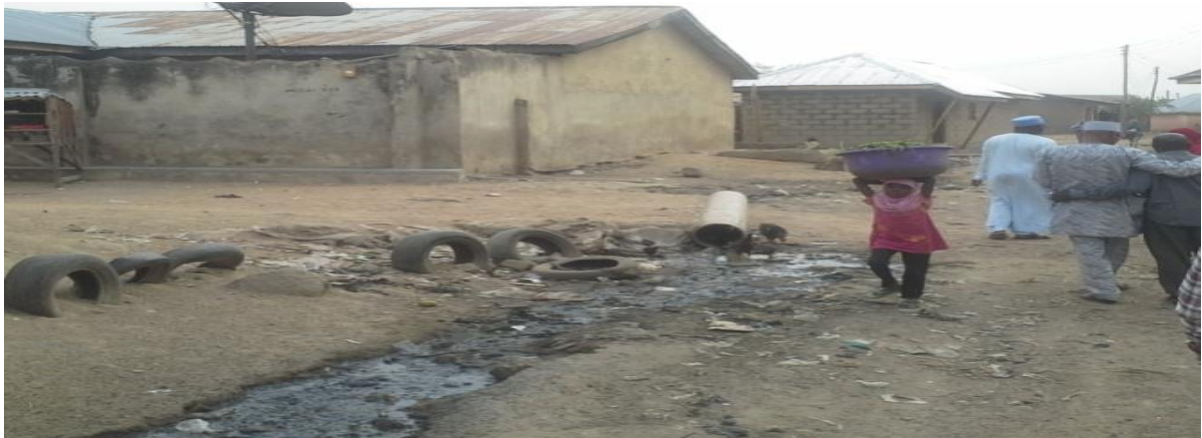
Plate I: Unplanned drainage cutting through the road Barkin-Sale area of Niger State, Nigeria Source: Author's fieldwork 2013
