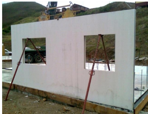
Figure 4: Erection of GFRG panels over plinth beam at site
