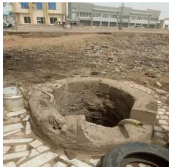
Plate 2: Well located at filthy (Defecated)
