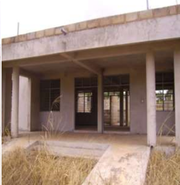
Figure 4: The Senior High School (under construction)
