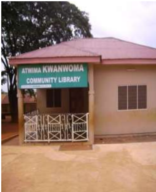
Figure 3: The Community Library (under construction)
