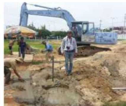
c. SCPile after drilling
