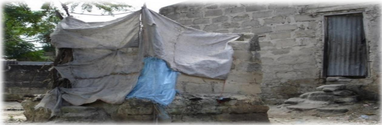
Plate 2.1: A typical pit latrine
