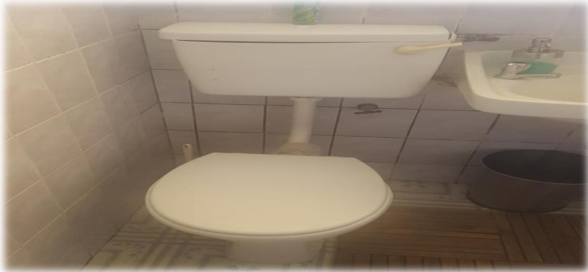
Plate 2.4 Conventional cistern-flush toilet
