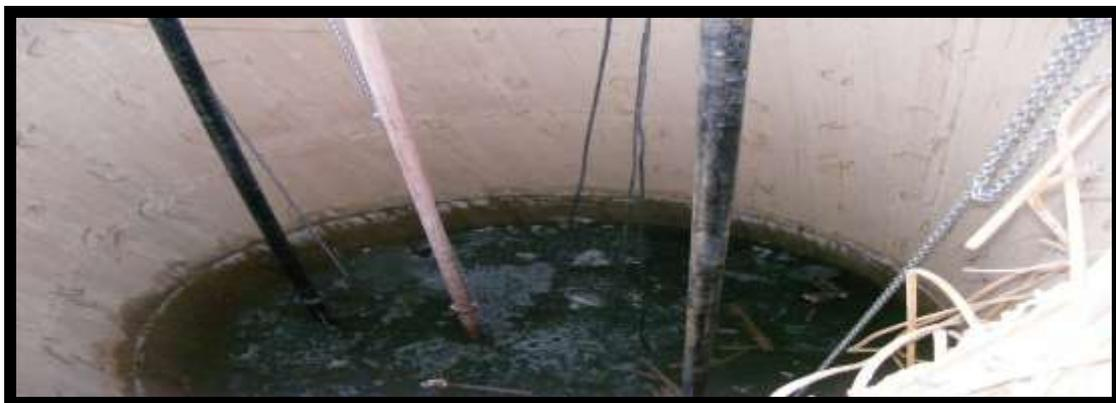
**Figure (6)** A photograph of the large diameter well and the four submersible pumps.
