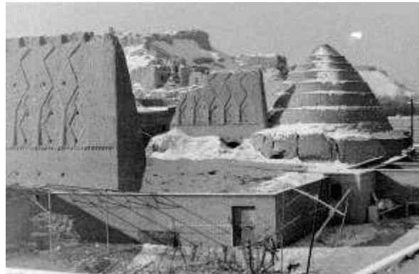
Figure 1: ZARSIF refrigerator in Kerman city. Iran Source: Documentation Centre of the Faculty of Architecture and Urban Planning, Shahid Beheshti
