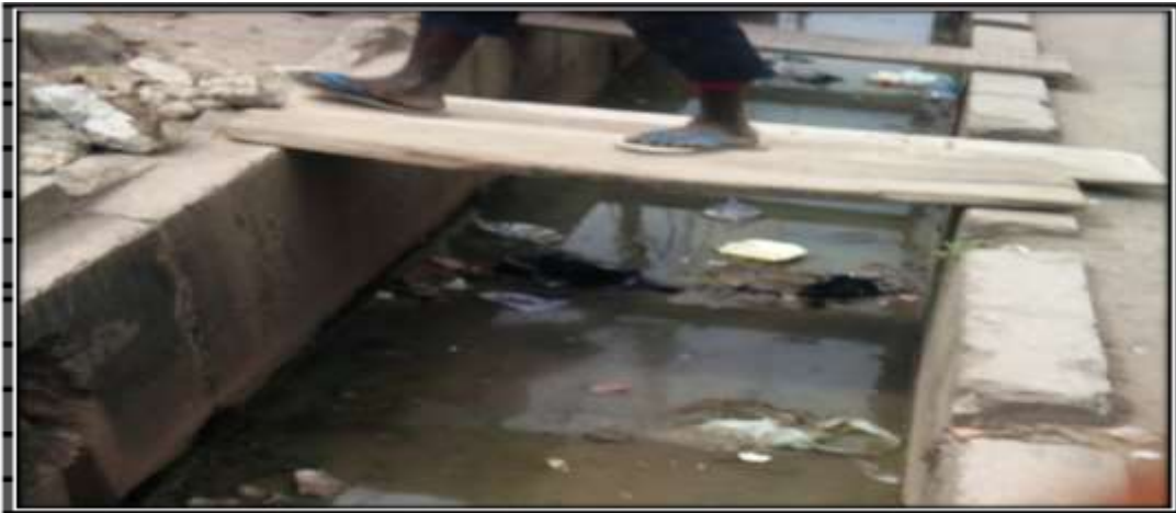
Plate 2 Disposed sachet water in gutter along Kodesho Road, Ikeja.
