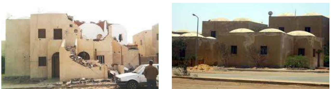
Figure (8) low cost construction system in orascom low-income housing
