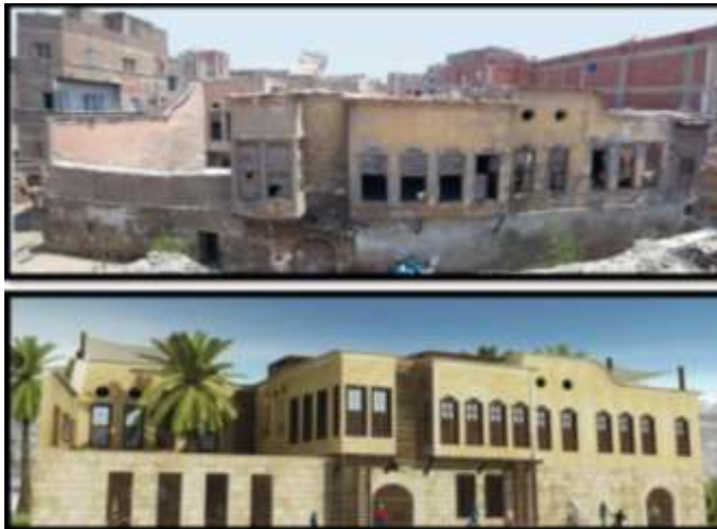
Figure 23: Building façade before and after development, in that order
