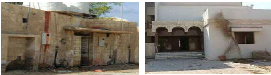
Figure 18: Abandoned buildings demolition operation, Al Sharqa Municipality, U.A.E.
