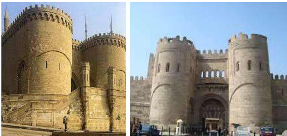
Figure 15: Bab Al Gharb, an example of closed historic sites in Egypt
