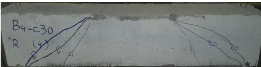
Figure (8) Crack Pattern of Beam (B4)
