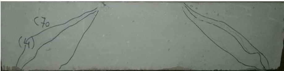
Figure (10) Crack Pattern of Beam (B6)
