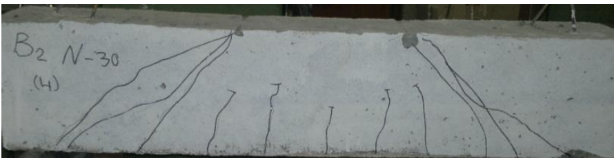
Figure (6) Crack Pattern of Beam (B2)
