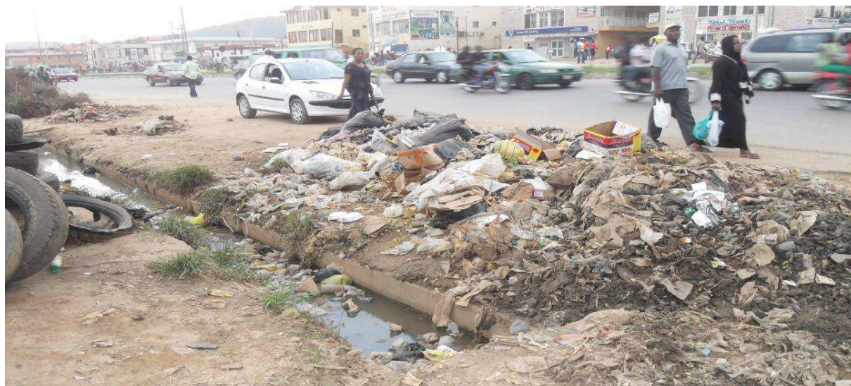
Figure 12: A Heap of mixed garbage removed from a blocked drainage channel along Abuja-Keffi Expressway, near Sharp Corner – Mararaba.
