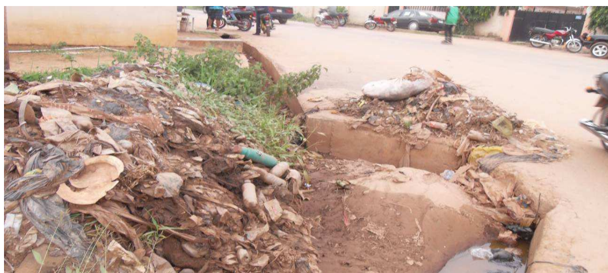
Figure 11: A heap of mixed solid wastes removed from a blocked drainage channel on the popular Abacha Road, Mararaba.
