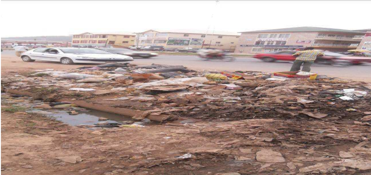
Figure 13: Another heap of mixed garbage removed from a blocked drainage channel along Abuja-Keffi Expressway at another location at Mararaba.
