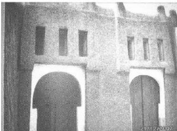
Figure 11: Entrance of Hausa building showing “Zanko”
