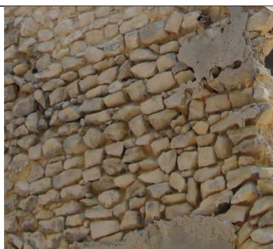
Figure 7: Deteriorated joint mortars resulting from soft and friable mortar
