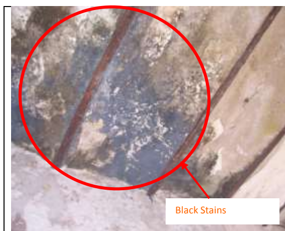
Figure 8: Condensation and black mould and stains growth on the walls
