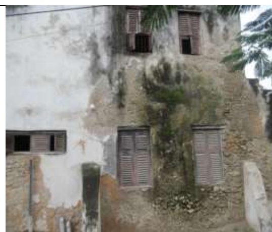
Figure 9: Fungi Attach on the Walls of Old Fort resulting from exposure to environmental agents
