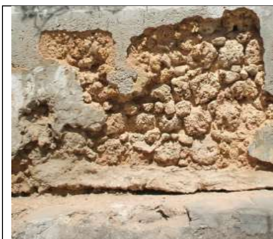
Figure 6: Peeling off plaster as a result of the use of soft and friable mortar
