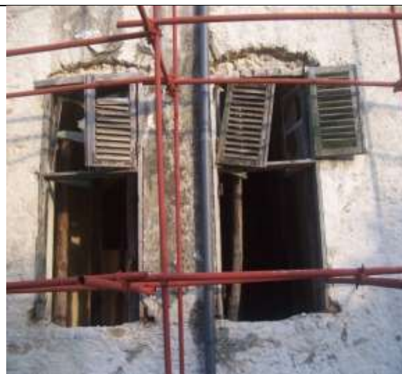
Figure 2: Deteriorated Windows
