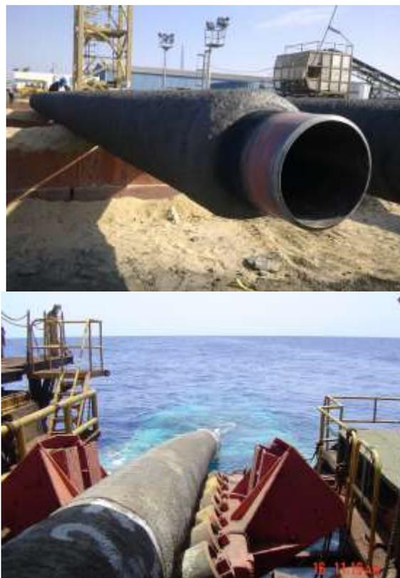
**Fig. 1: Concrete Weight Coating (CWC) for offshore pipeline**
