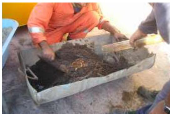
Preparation concrete mix (hematite-barite ore, sea water cement & water)
